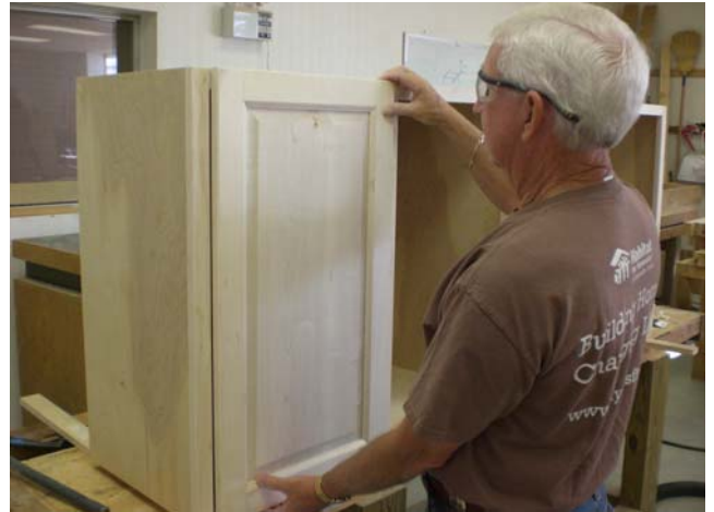
Bill Bagwell test fits raised panels for one of the classroom storage cabinets
